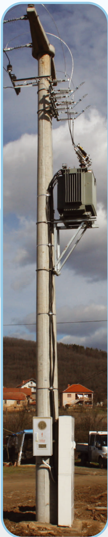
Measuring distribution box with fuse rails for pillar transformer 10 / 0,4 kV
