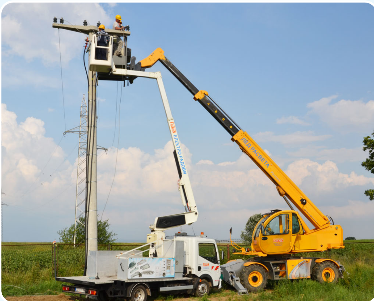
PART OF MACHINERY FOR CARRYING OUT WORKS ON NETWORKS 0,4, 10, 20 AND 35 KV
