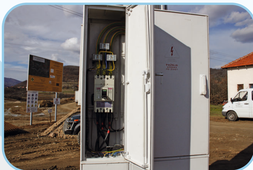
Measuring distribution box with fuse rails for pillar transformer 10 / 0,4 kV
