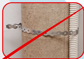
Correct and incorrect placing a flexible hose on the pillar
