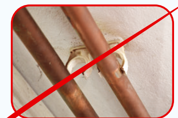
Correct and incorrect placing copper pipes for heating
