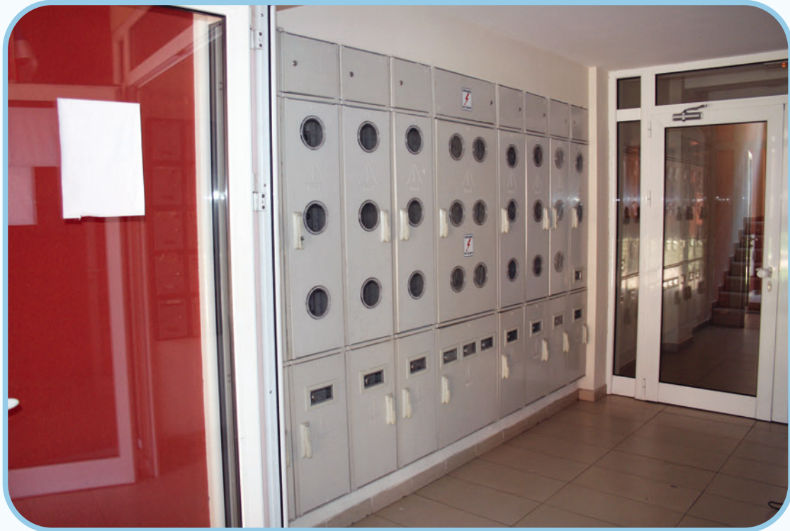
Polyester modular cabinet for 27 measuring points
