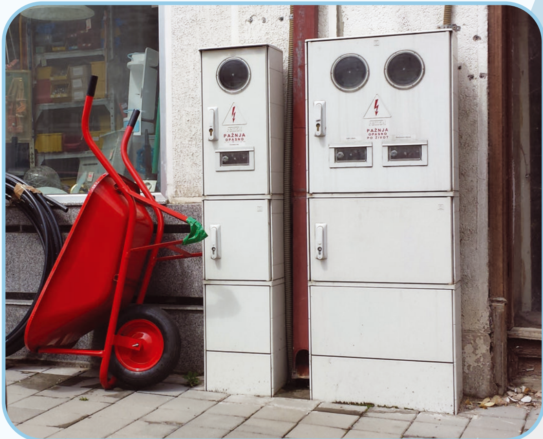
Stand-alone grounding cabinet for 1 and 2 measuring points
