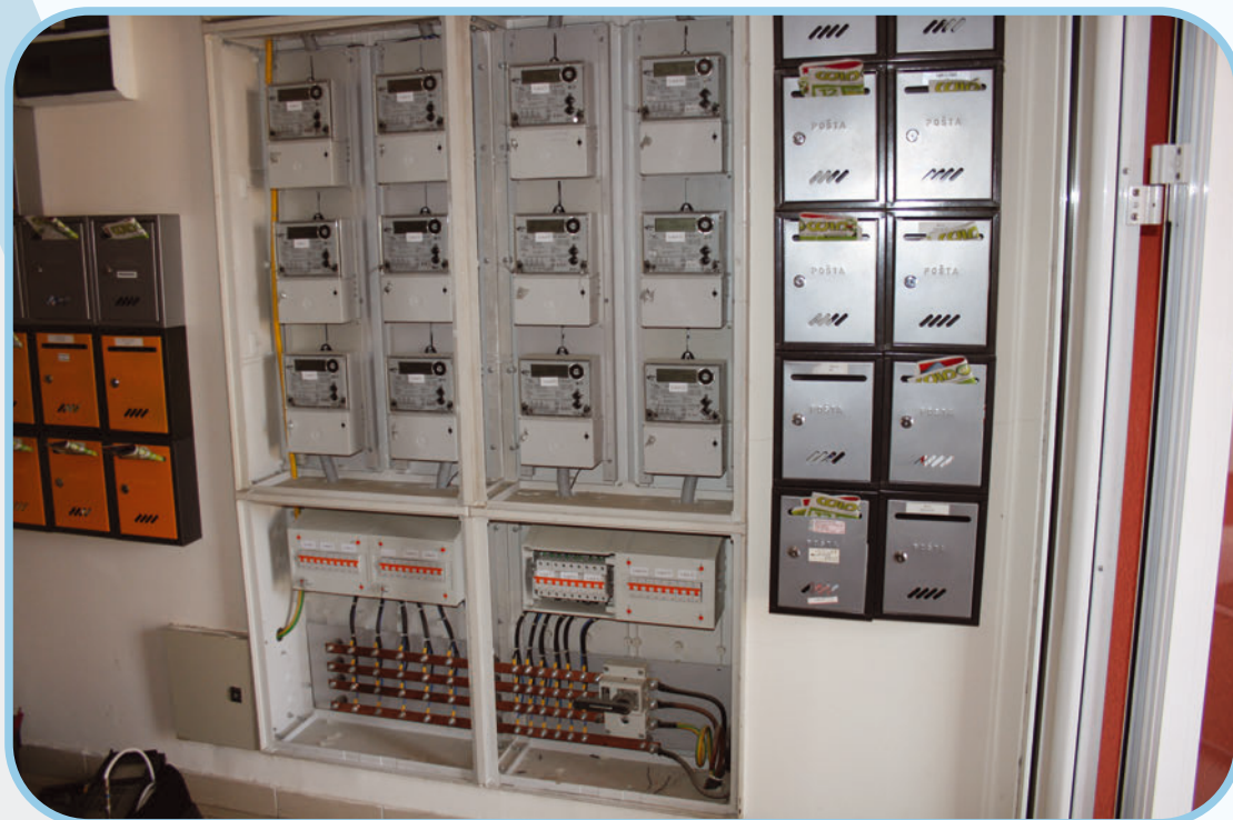
Polyester modular cabinet for 12 measuring points
