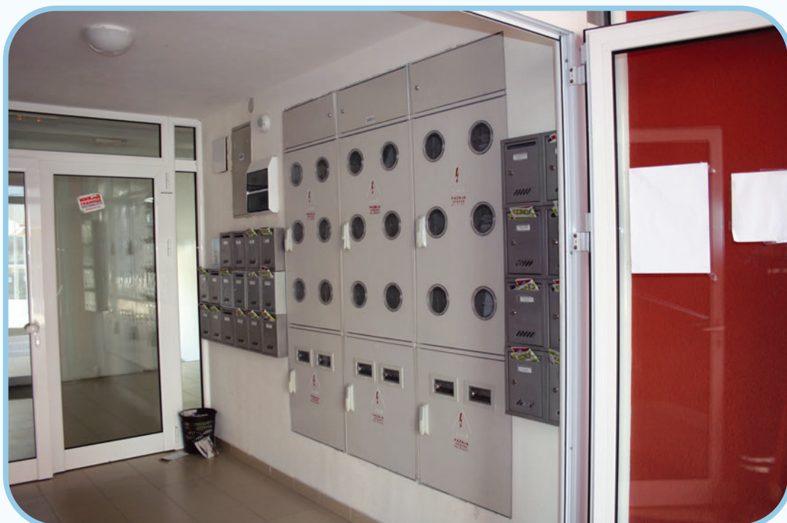
Polyester modular cabinet for 18 measuring points
