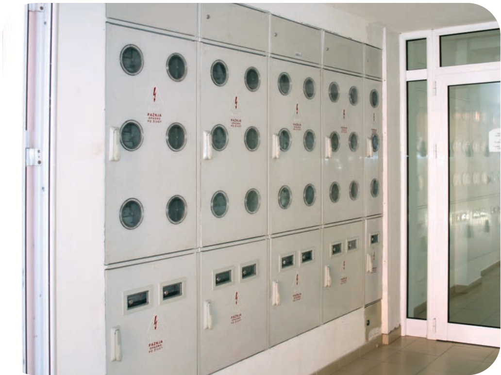
Note: Designed for the installation of meter mounting boards with dimensions of 220x330 mm.
